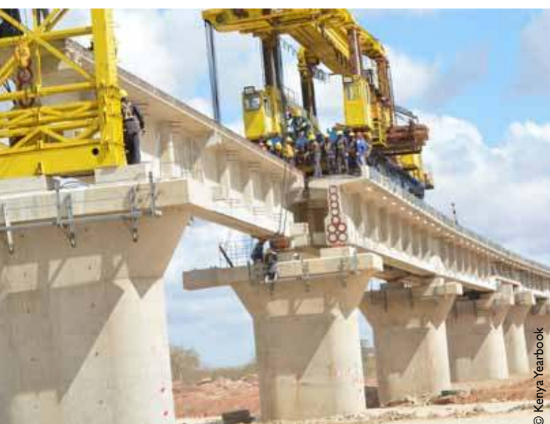
Construction of Standard Gauge Railway in Kenya
